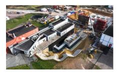
01/04/2024 To the west, the southern embankment of  $S^3$  is reconstituted to a depth of -3.5 m, thus definitively burying the -3 and -2 levels of DESIR. To the east, the veil of the experimental hall gradually rises to its final height of 12 m.
