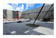
30/06/2024 Installation of the first welded reconstituted beams (30m, 11t), which will support the hall roof and enable the building to meet its static and seismic structural requirements.
